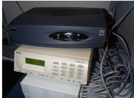
Ad Tran TSU 120 CSU/DSU and Cisco 1700 Series Router
